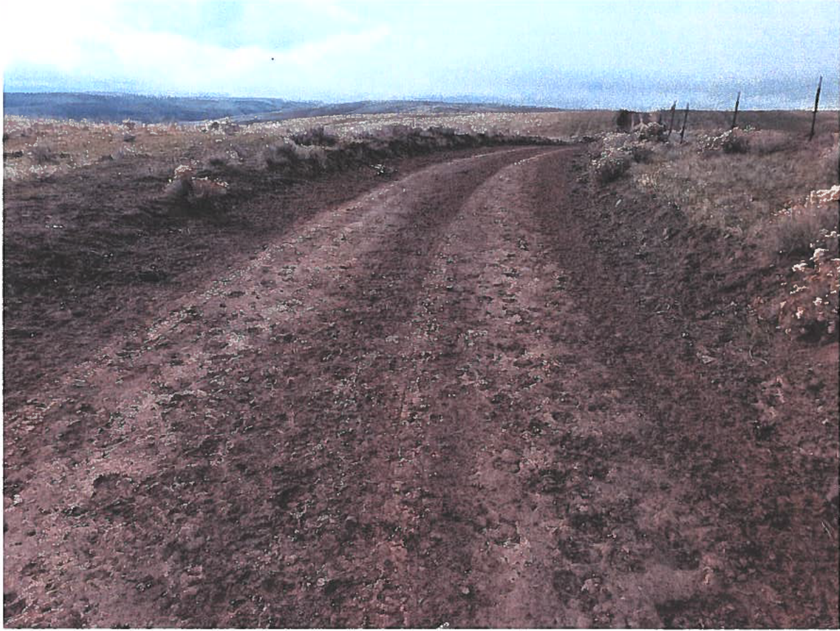
B. Hammel – Haul Road Before Photos
